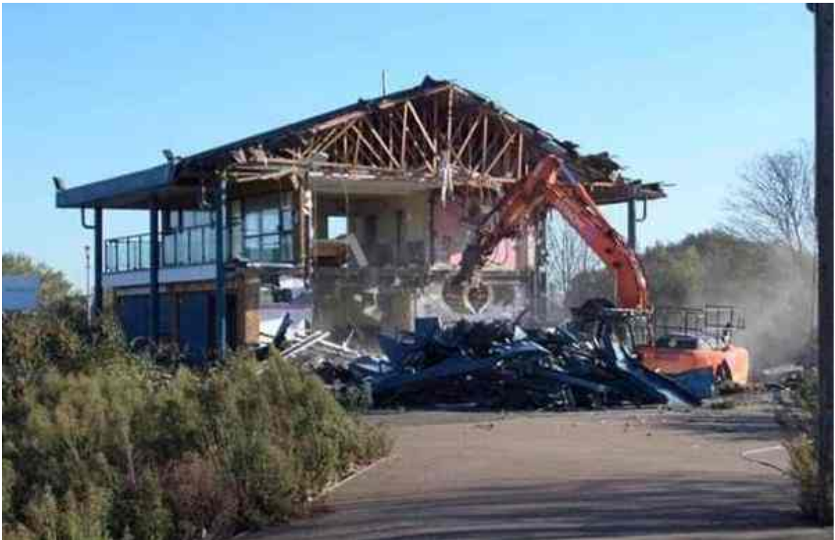
The Raceway Tavern under demolition, Arena Essex, November 2020. This is the photograph, then circulating online, which was sent to Thurrock Council on 10 November 2020 and which prompted planning enforcement case 20/00442/AUNWKS.
